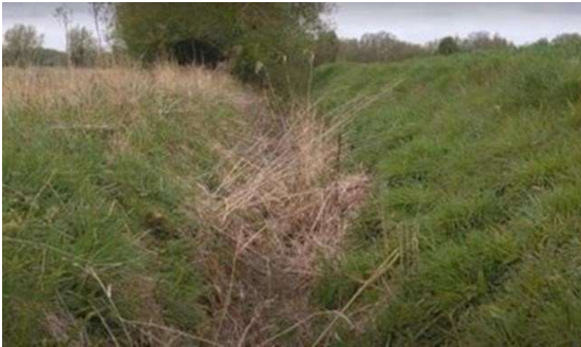
Photo 1 Existing ditch along northern boundary of Work Area 39
